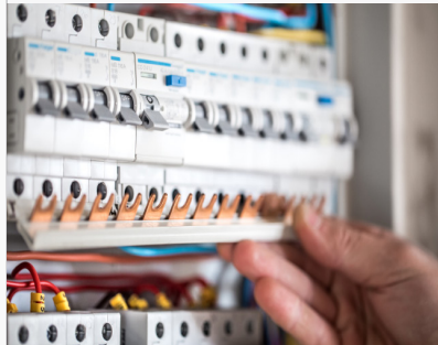
Electrical Equipment Installations
